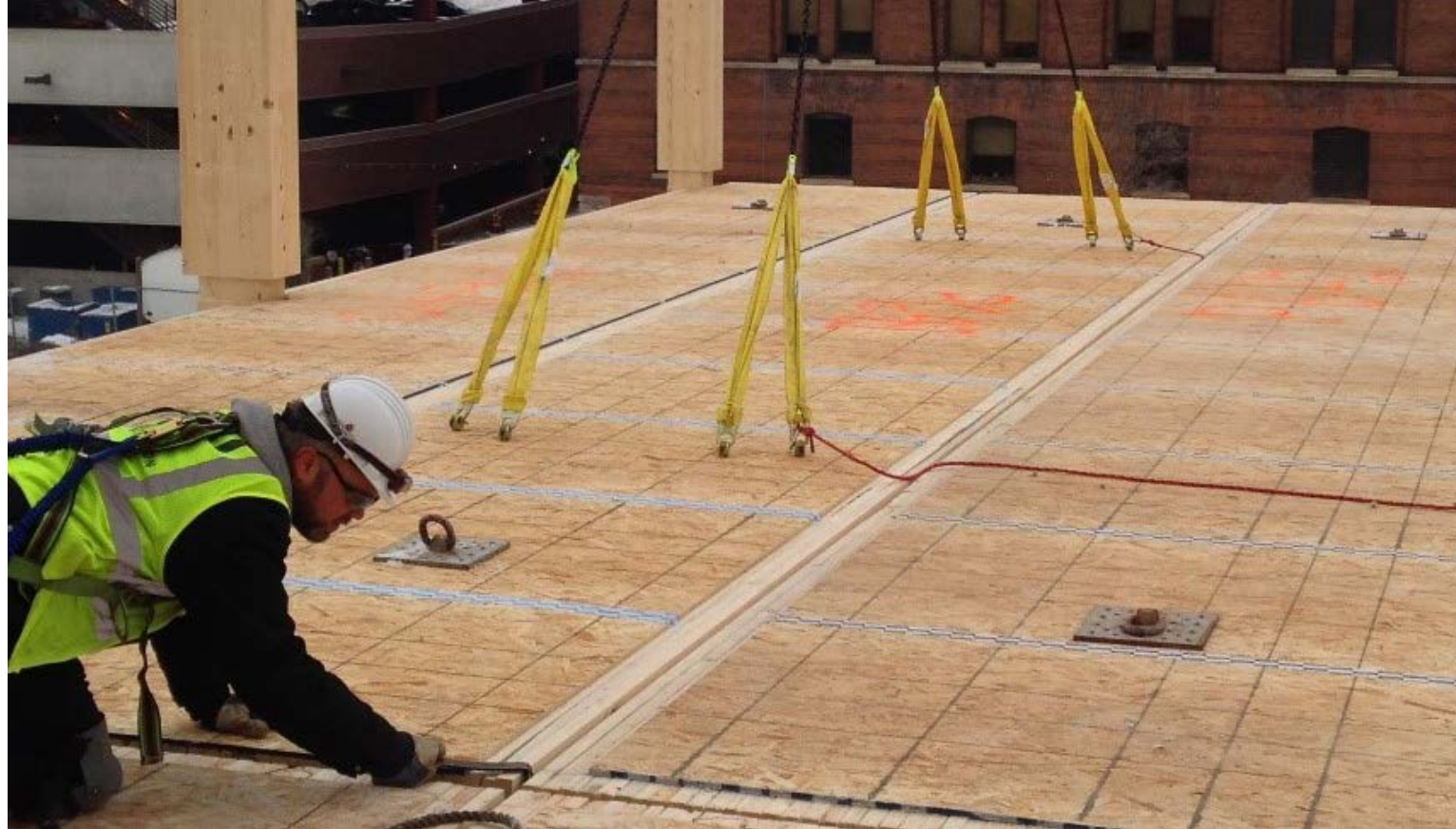
Figure 8.4 Installed roof panels with gaps for expansion Photo courtesy of StructureCraft
