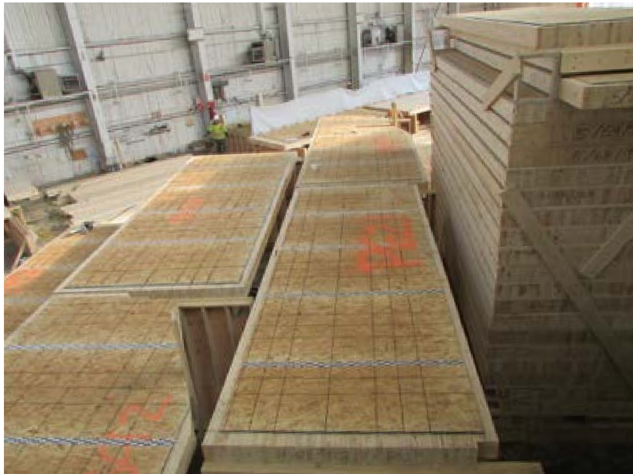
Figure 8.2 Storage setup with dunnage and stickers Photo courtesy of StructureCraft
