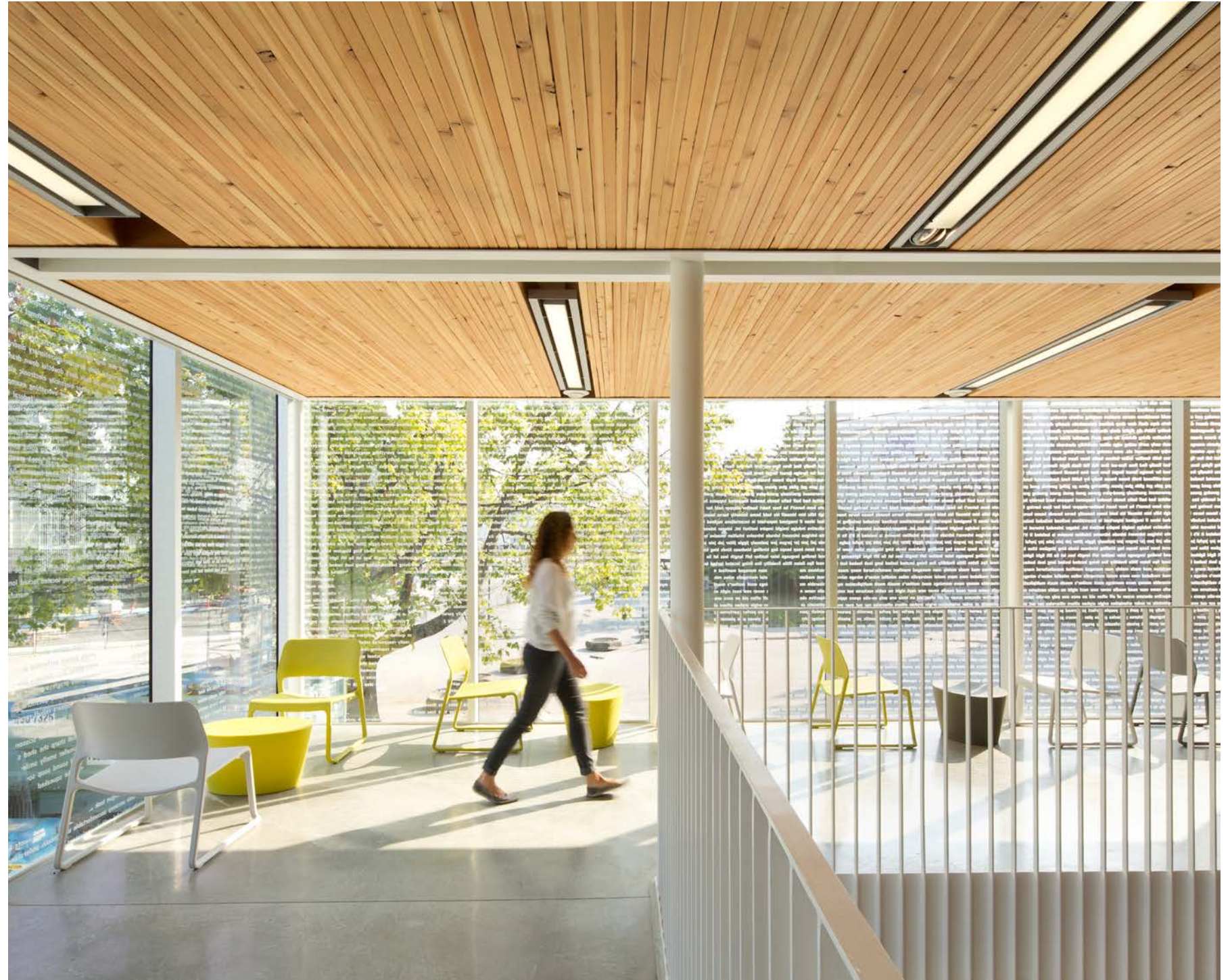
Below Architectural grade NLT shown at UBC Bookstore, Vancouver, BC Photo credit Ema Peter Photo courtesy of Fast + Epp
