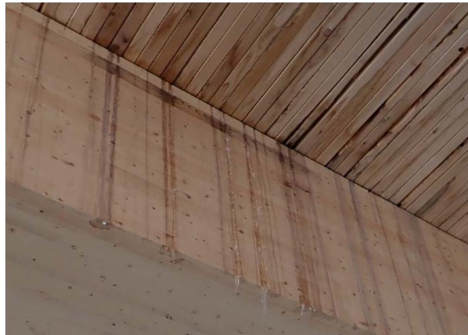
Left | Figure 8.6 NLT exposed to excess moisture during construction. Wetting occurred on the NLT between laminations and staining on the NLT and structure below. Water dripping on the underside of the panel and beam froze and formed icicles. Photo courtesy of RDH Building Science
