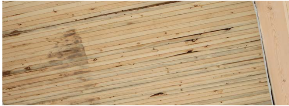
Figure 6.1 NLT Showing blue staining from beetle-killed wood Photo courtesy of Perkins&Will
