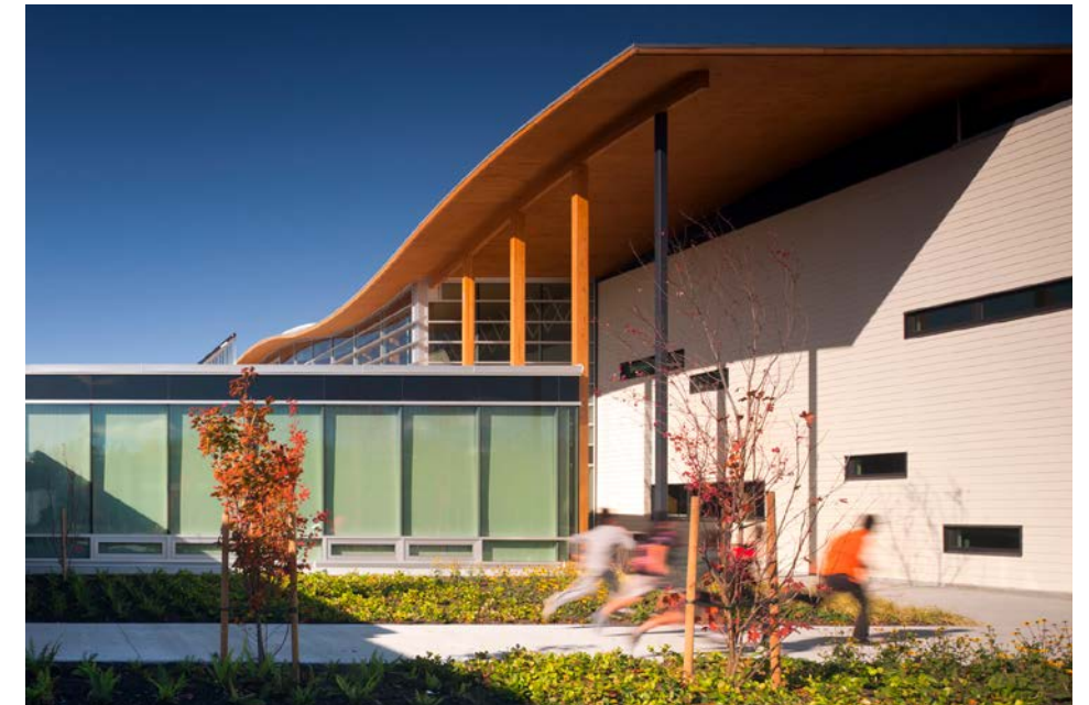
Figure 2.13 Example of continuous soffit from interior to exterior. Samuel Brighthouse Elementary School, Richmond, BC Architecture by Fast + Epp Photo credit Nic Lehoux
