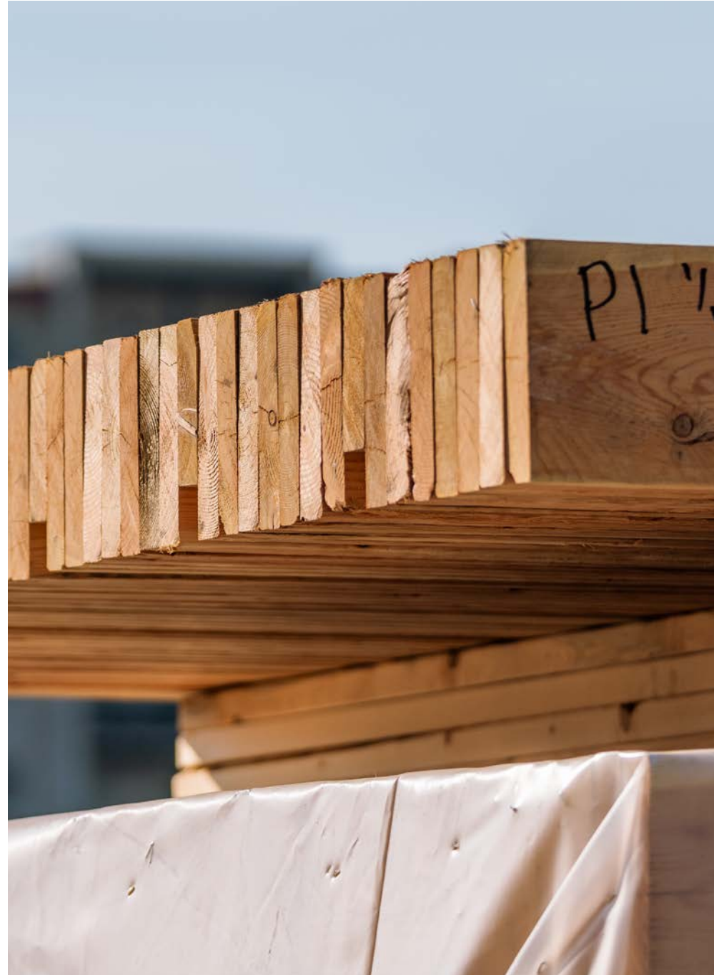
Figure 8.9 Exposed end grain edge of NLT panel Photo credit Bryce Byrnes Photo courtesy of NaturallyWood
