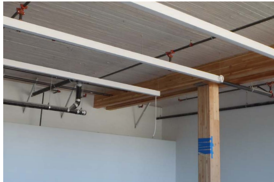
Figure 2.12 Office partition walls in Head Office, Vancouver, BC Photo courtesy of Fast + Epp
