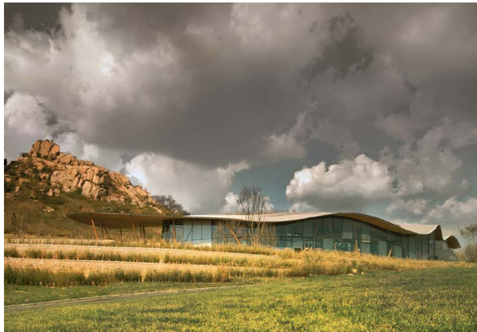
Figure 2.6a Freeform curvature with NLT, Tsingtao Pearl Visitor Centre, Qingdao, China Architecture by Bohlin Cywinski Jackson Photo credit Nic Lehoux
