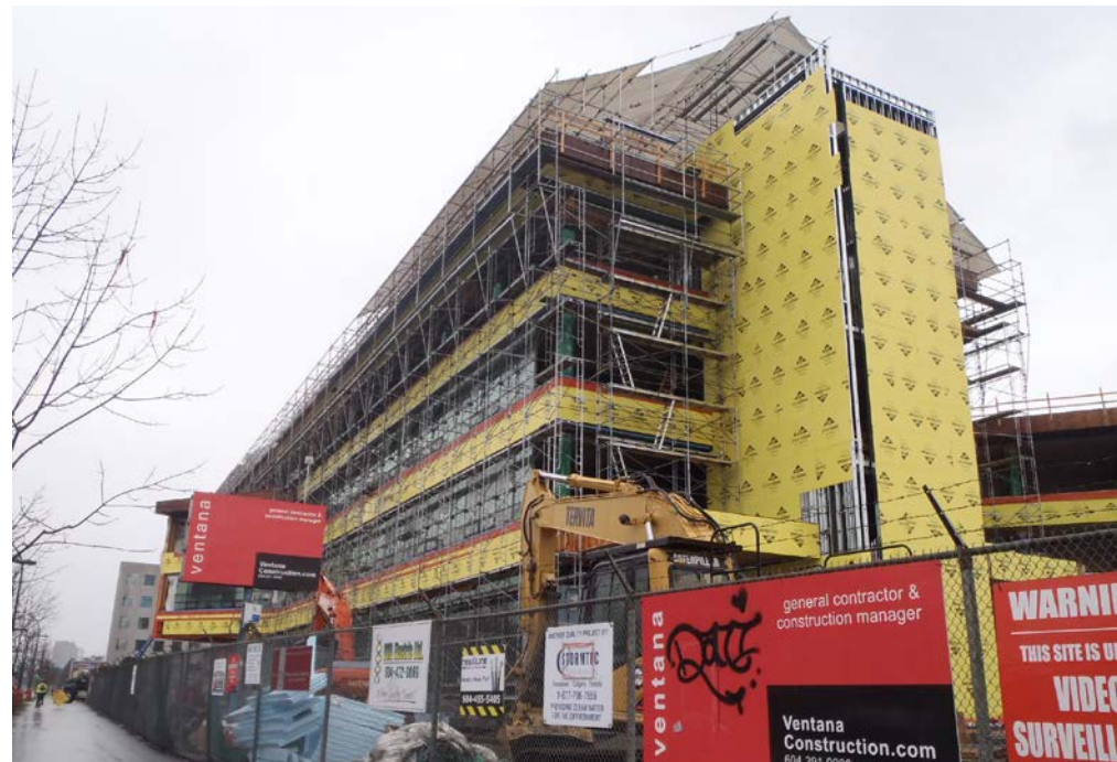
Figures 8.13 Fixed tenting installation Photos courtesy of Fast + Epp
