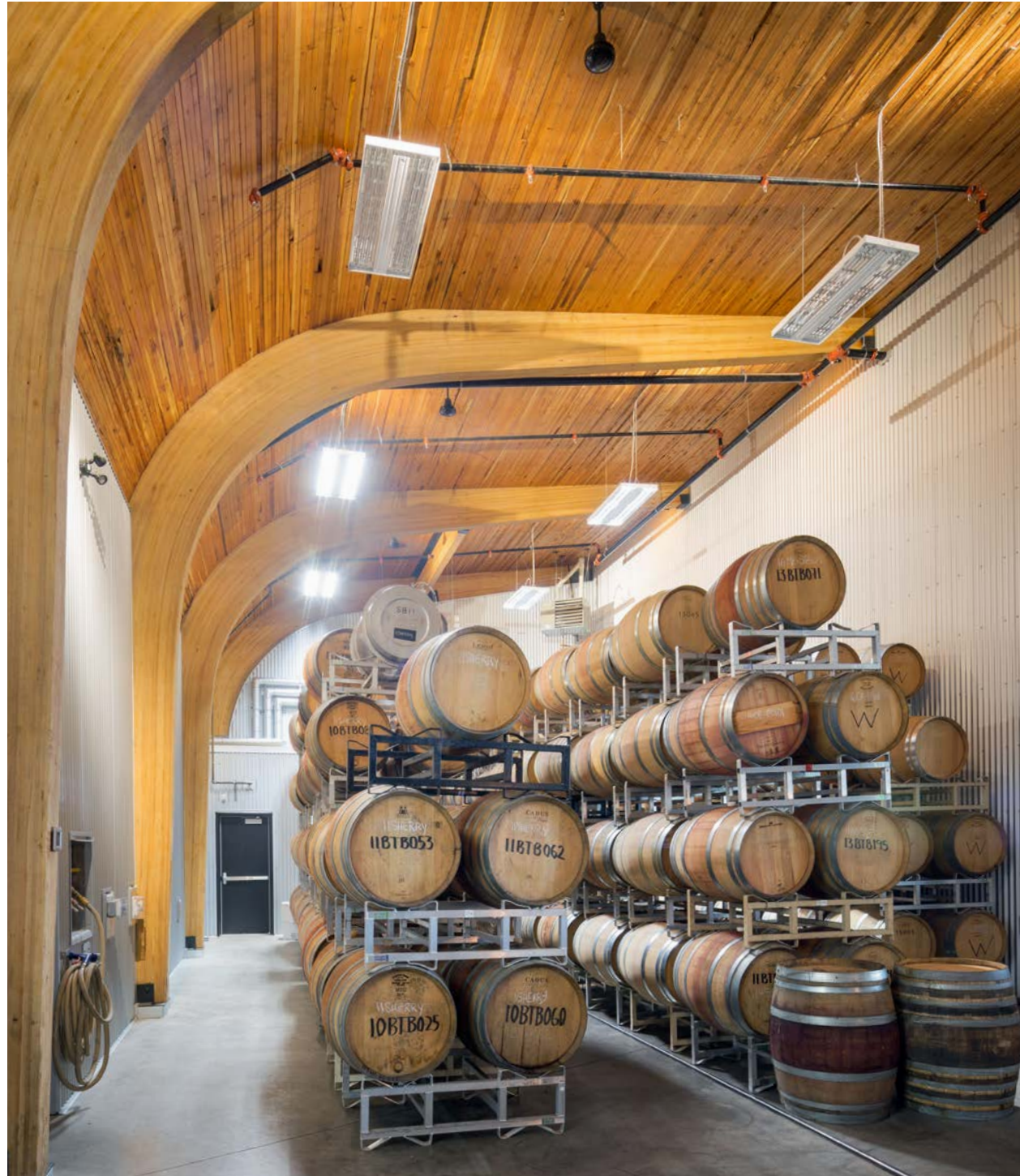
Below Industrial grade NLT shown at Time Winery, Kelowna, BC Photo credit Dan Schwalm Photo courtesy of HDR
