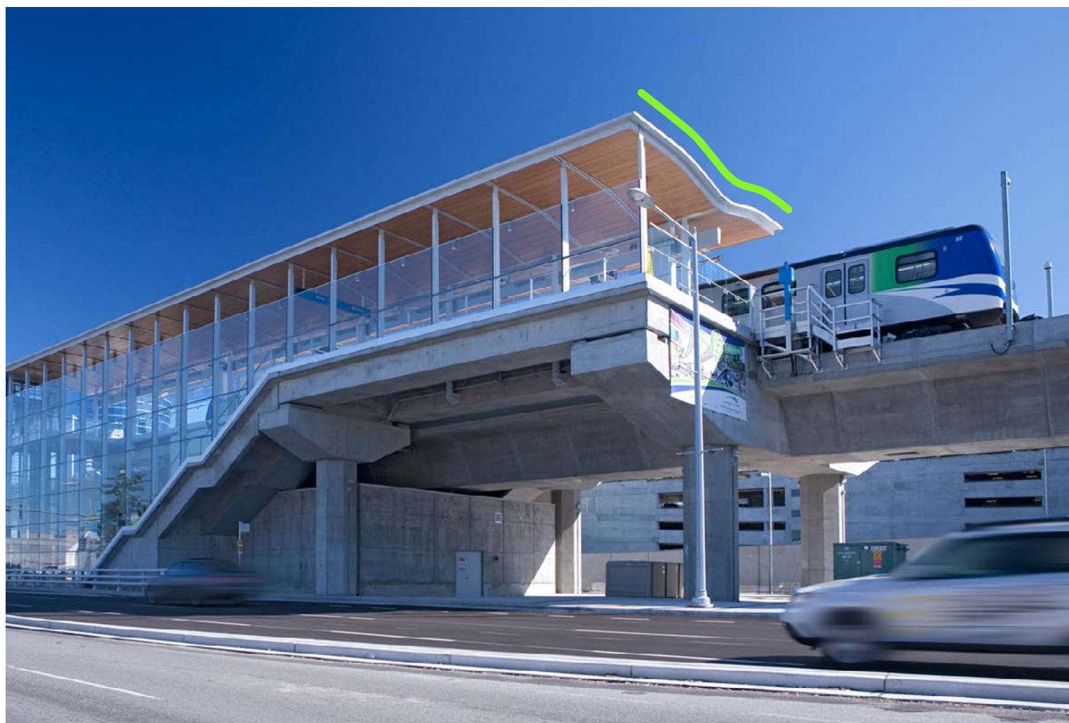
Figures 2.3 NLT on curved steel channels, Aberdeen station, Richmond, BC Architecture by Perkins&Will Photo courtesy of Perkins&Will
