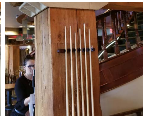
Figure 3.11 Structural connection with column cap at the Landing Building Photo courtesy of GHL Consultants Ltd.
