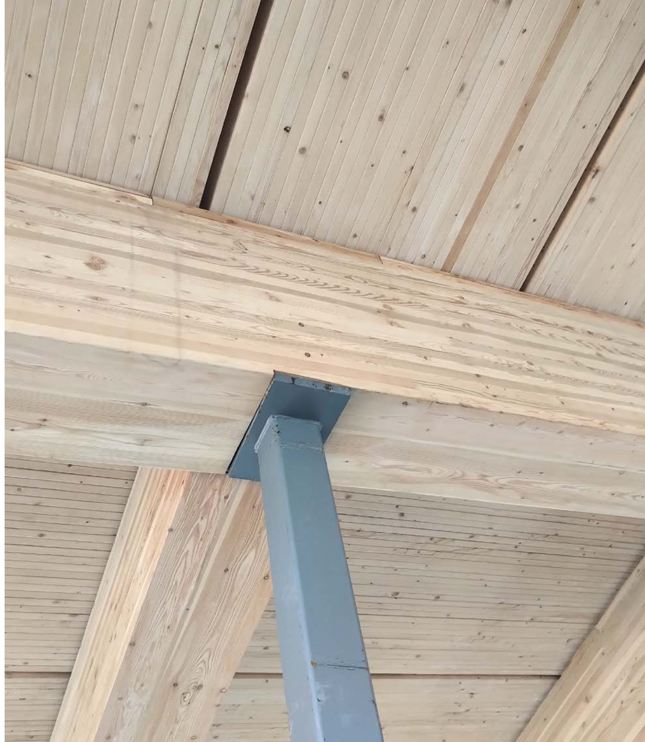
Below Premium architectural grade shown at Ādisōke Public Library, Ottawa, ON Architecture by Diamond Schmitt Photo courtesy of Fast + Epp
