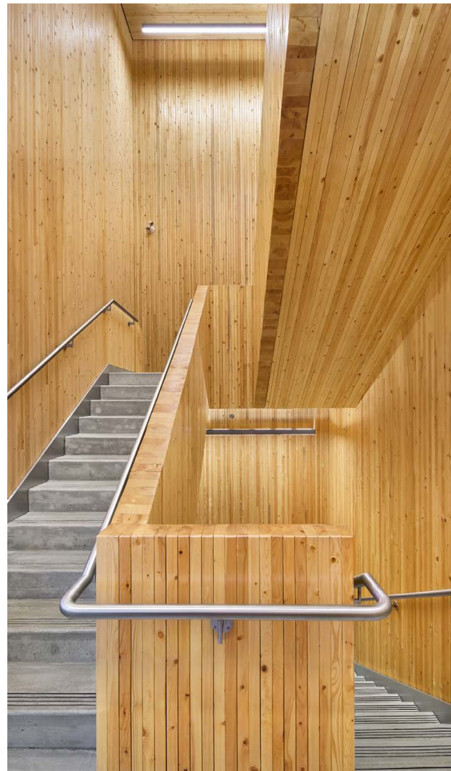
Figure 2.2 NLT Stair at Prince George Fire Hall No 1, Prince George, BC Architecture by hcma Photo credit Ed White Photographics Photo courtesy of NaturallyWood
