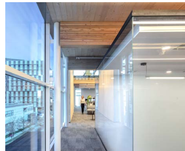
Figure 3.10 Timber floor steel column Photo courtesy of Fast + Epp
