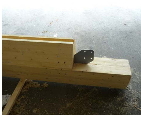
Figure 3.8 Internal steel plate connection buried within wood member Photo courtesy of FPIinnovations
