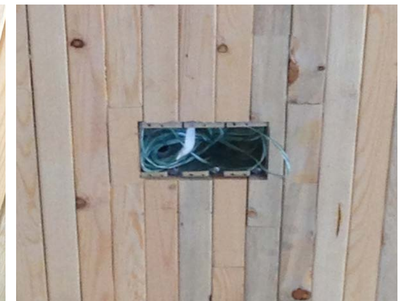
Figure 2.15b NLT panel after capping the service chase Photo courtesy of StructureCraft
