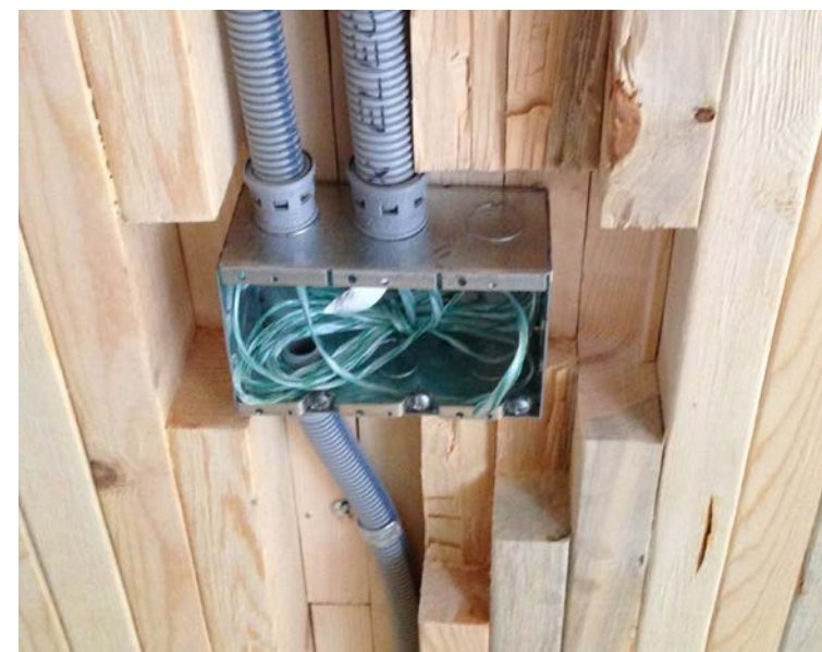
Figure 2.15a NLT panel before capping the service chase Photo courtesy of StructureCraft
