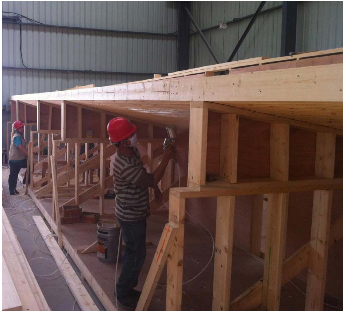
Figure 7.4 Shop applied coating on NLT
