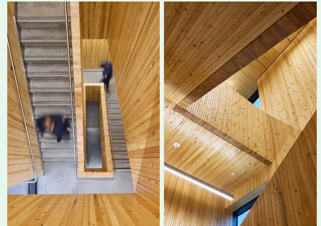
Above Prince George Fire Hall No. 1, Prince George, BC Photo courtesy of hcma Photo credit Ed White Photographics
