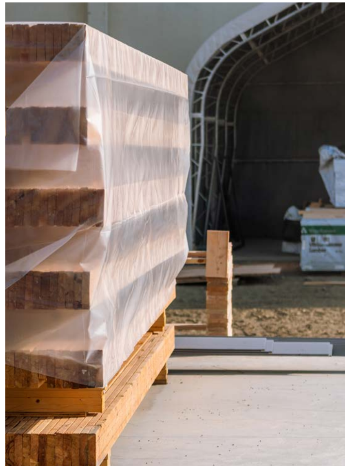
Below Storing NLT panels Photo credit Bryce Byrnes Photo courtesy of NaturallyWood
