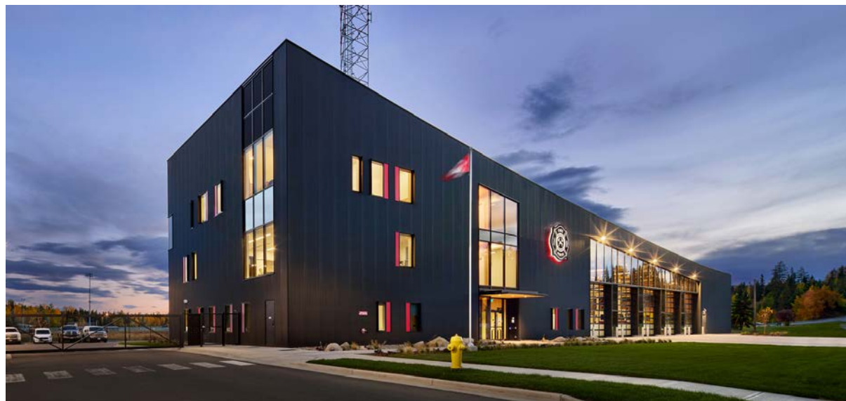
Below Prince George Fire Hall No.1, Prince George, BC Architecture by hcma Photo credit Ed White Photo courtesy of NaturallyWood
