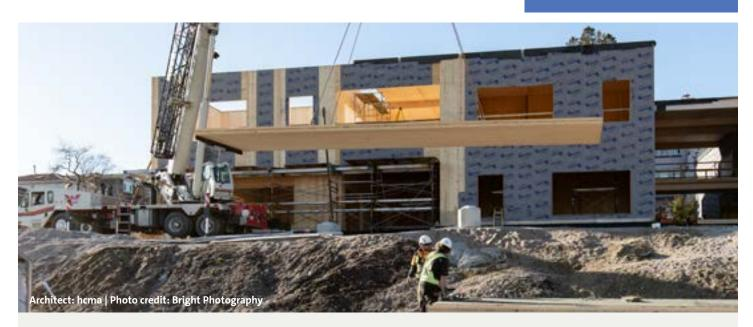
Long-spanning mass timber forms the school's quadrant configuration of Sir Matthew Begbie Elementary School in Vancouver. Cross-laminated timber (CLT) serves as both gravity and shear walls, to resist the high seismic forces of the region. CLT and connectors were fabricated off-site and delivered to site for easy erection.
