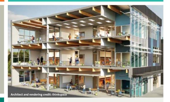
Ta'talu Elementary School, in Surrey, will be the first three-storey hybrid mass timber elementary school in BC when completed in 2024. The predominant structure will be post-and-beam glulam, with light wood framing. Load bearing members (beams and columns) will be mass timber. Mass timber was chosen because it matched the school's sustainability ambitions to reduce carbon emissions—adding to the aesthetic, biophilic, and enhanced learning properties that wood offers.
